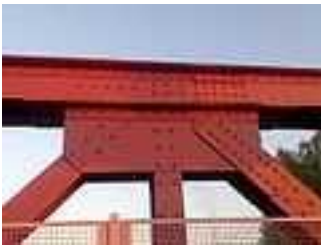
Figure 6.2 Member connections (from Wikimedia Commons)
