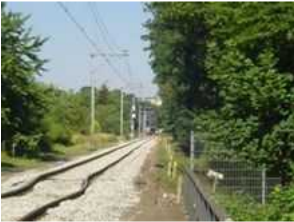
Figure 9.2 Buckling of tracks (Wikipedia)
