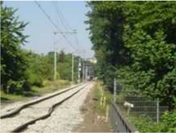
Figure 3.12.2 Buckling of tracks (Wikipedia)
